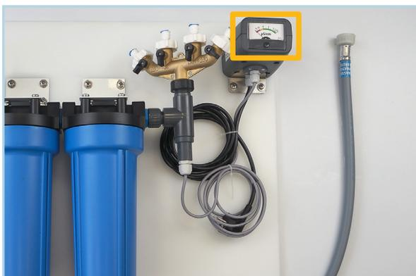
There is a conductivity meter mounted on the water filtration system. If the pointer of the display is in the green area ( $<10 \mu\text{S}/\text{cm}$ ), everything is in order. If the value is  $>10 \mu\text{S}/\text{cm}$ , the de-ionizer cartridges need to be replaced.
